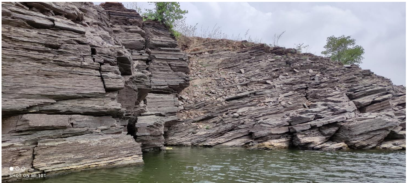
Figure 3.3: Photograph showing rock exposure and steep relief of ground noticed close to waterline
