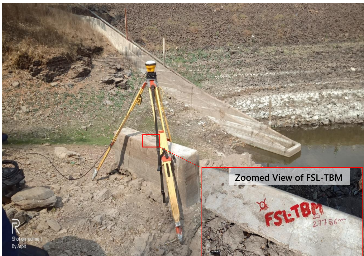
Figure 3.1: Machhannala Dam Benchmark (FSL-TBM)
