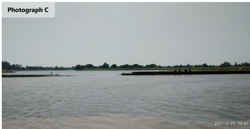
Photograph C: Southernmost approachable part of the Machhannala Reservoir (413663 mE, 2547271 mN) with partially submerged section of road and shallow water depth.
